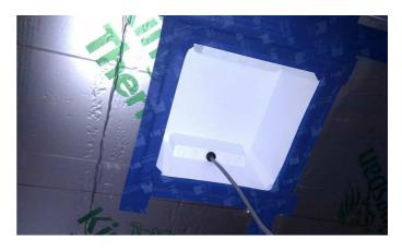
• **FF Perimeter** of Floor must be sealed. The 300mm deep Floor Void is a massive risk. If the airtight detail isn't correct or leaks any air (between floors to external wall) then the whole void becomes a potential risk.
