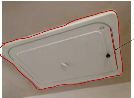
Install good quality trapdoors fitted with airtight seals. Trap-doors & Loft Hatches cannot be taped for the duration of the airtest. Have you taped the joints of the insulation? This can make a great difference to the airtightness of the property.
