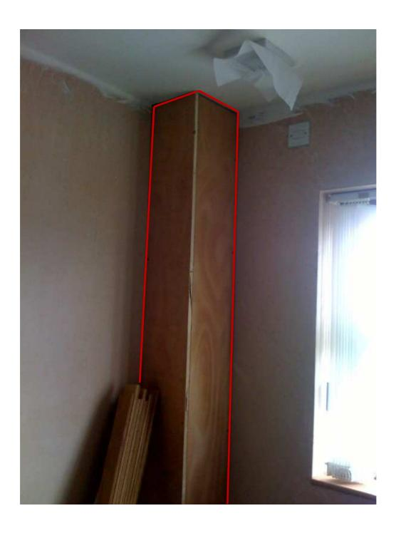
• Be Careful if Boiler Flue is boxed in as it is never usually airtight around the flue hole behind the facing board
